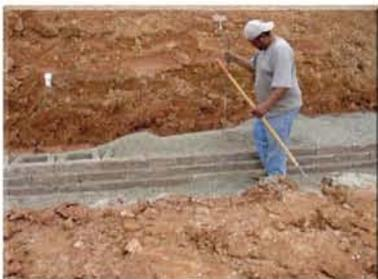
After core filling the block, use a rod to drive down into the cores to assure a thorough core fill. Backfill should be level to top course of block.
