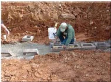
When laying the first course, level the block front to back and side to side with a two foot carpenter's level. It is very important that the first course be level and placed on a compacted footing.
