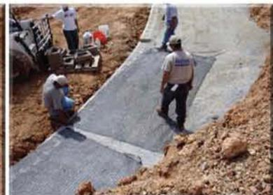
Next lay out the geogrids. Their length will depend on the wall height. Rule of thumb is no less than 75% of wall height (no shorter than 4') and no less frequent than every 2 vertical feet.
