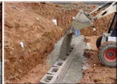
It is recommended that the cores of the block be filled with a #67 or #78 stone no less frequently than every three courses. This same stone is recommended for the backfill as well.
