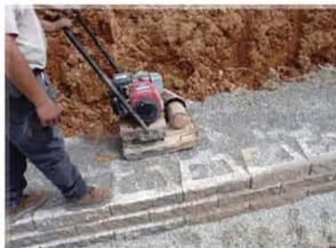
Compacting the backfill is very important. This provides additional resistance to pressures exerted on the wall and prevents settlement. Repeat this process after each backfill.
