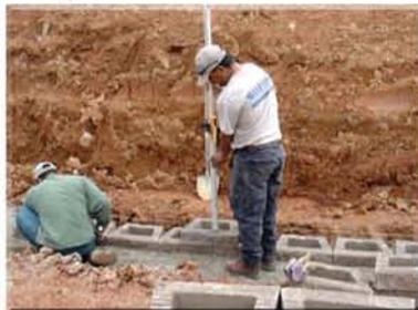
It is always a good idea to shoot grades from time to time to ensure your wall is maintaining the correct level.
