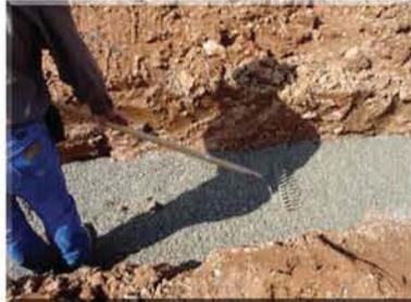
The footing depth will vary based on the height of the wall. Rule of thumb is 1 inch of embedded block per vertical foot of wall height is required. Place four to six inches of crushed rock (#78 or #8910) in the footing and level for the wall foundation.
