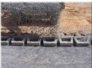
After laying out the grids, place another course of block down on top of the grids, align, then core fill and backfill. It is important that the grids be stretched tight prior to placing rock fill.
